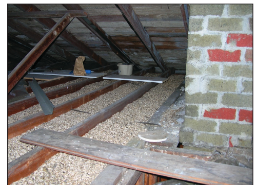
Typical vermiculite insulation in an attic
